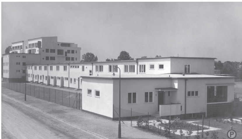
Fig. 21. The row houses by Effenberger et al. The flatness and uniformity of the block is apparent (Museum of Architecture in Wrocław).
