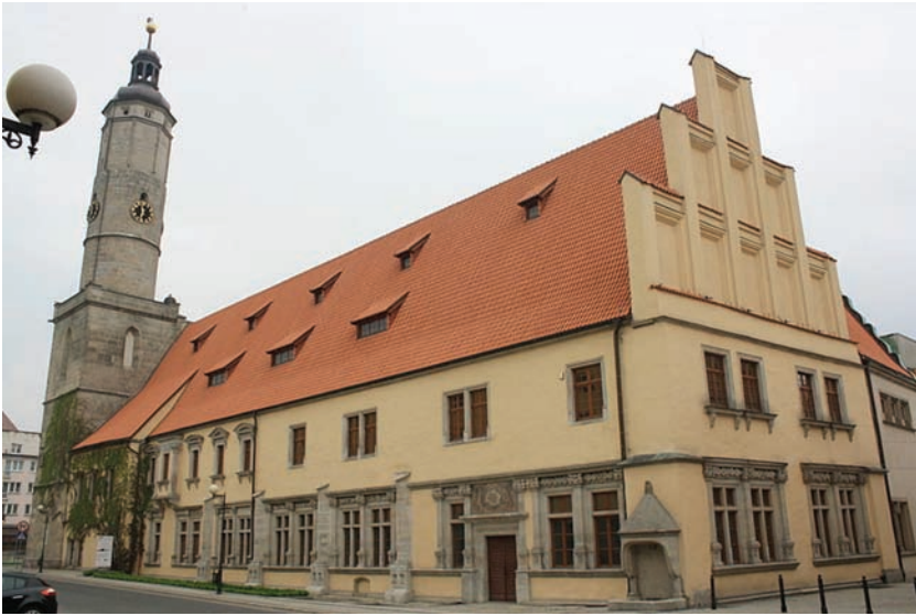
Fig. 31. Hans Poelzig renovated the Laski (Lowenberg) Town Hall. Contemporary photograph (Wikipedia image, courtesy of Oslm).
