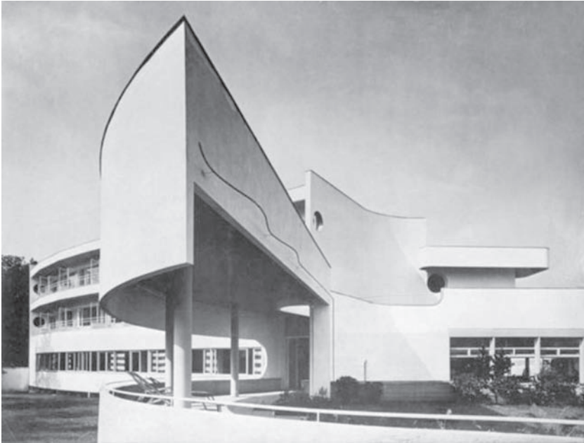
Fig. 27. Scharoun's Ledigenheim viewed from the garden side (Technical University Berlin).
