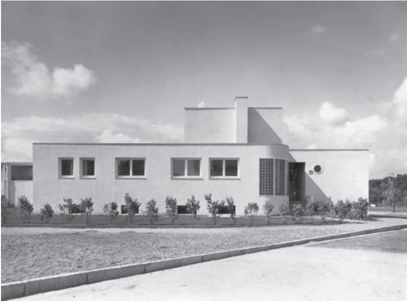
Fig. 23. Curved form and stepped massing at Lauterbach's House (Museum of Architecture in Wrocław).
