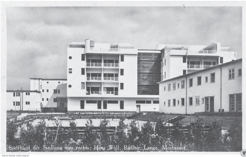
Fig. 26. Rading's Turmhaus . Originally planned to be eight stories it was only built up to the third. The animated facades featured windows of many sizes and shapes. (Museum of Architecture in Wrocław).
