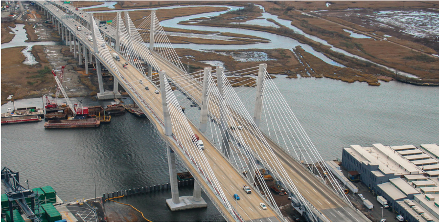
Fig. 7.6. The two spans of the new Goethals Bridge opened between 2017 and 2018. (Photograph reprinted by permission of Port Authority of New York and New Jersey.)
