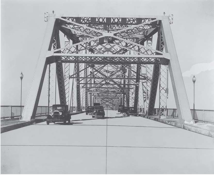
Fig. 7.3. Cars crossing the Goethals Bridge in the 1930s. ( Photograph reprinted by permission of Port Authority of New York and New Jersey. )
