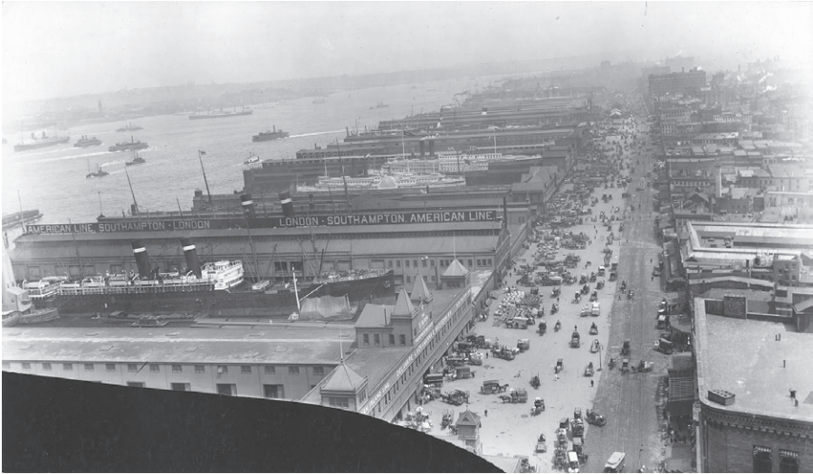
Fig. 2.3. Hudson River piers in Manhattan, c. 1905.
