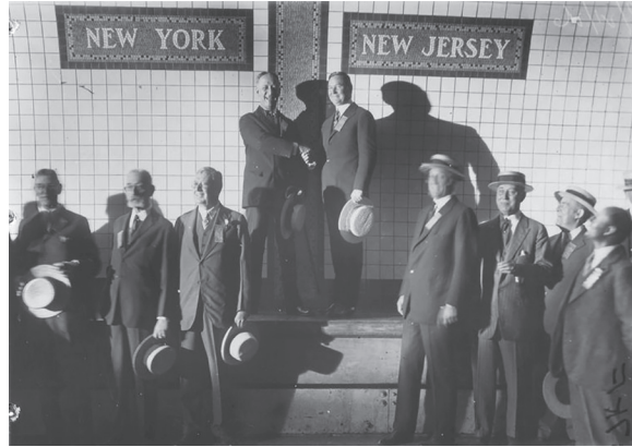
Fig. 2.6. Officials from New Jersey and New York shaking hands before the opening of the Holland Tunnel. (Photograph from the New Jersey Interstate Bridge and Tunnel Commission , courtesy New York Public Library Digital Collections .)
