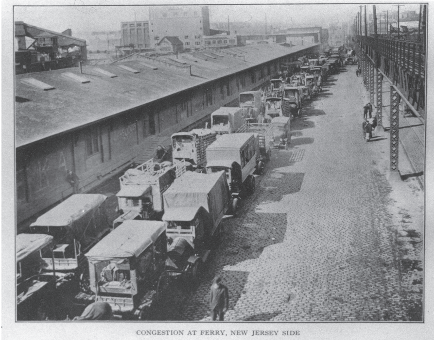
Fig. 4.1. Trucks lined up for the ferry in Hoboken (c. 1918–1919). (Photograph reprinted by permission of the Hoboken Historical Museum.)
