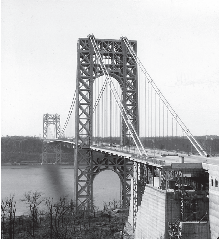
Fig. 2.7. George Washington Bridge under construction.
