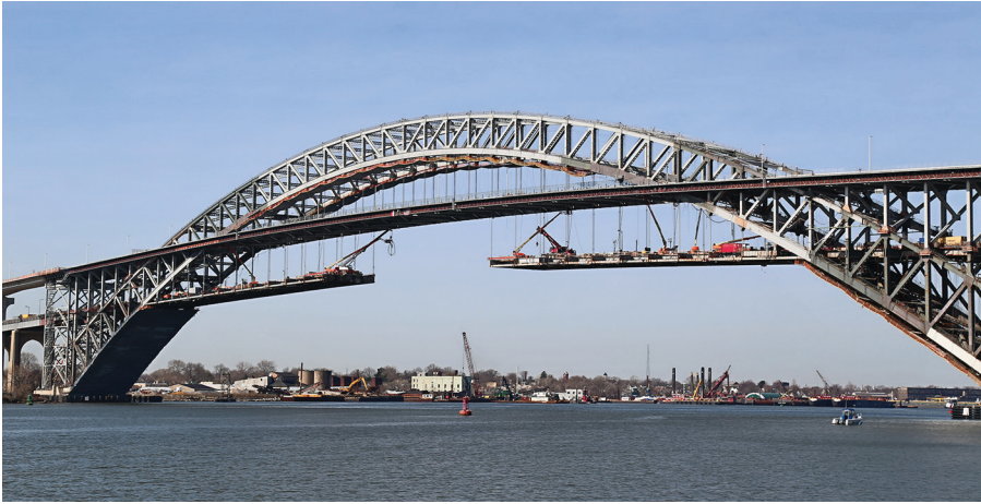
Fig. 7.8. Construction underway at the Bayonne Bridge to raise the bridge's clearance by sixty-four feet. The original deck has yet to be fully removed in this photo. (Photograph reprinted by permission of Port Authority of New York and New Jersey.)
