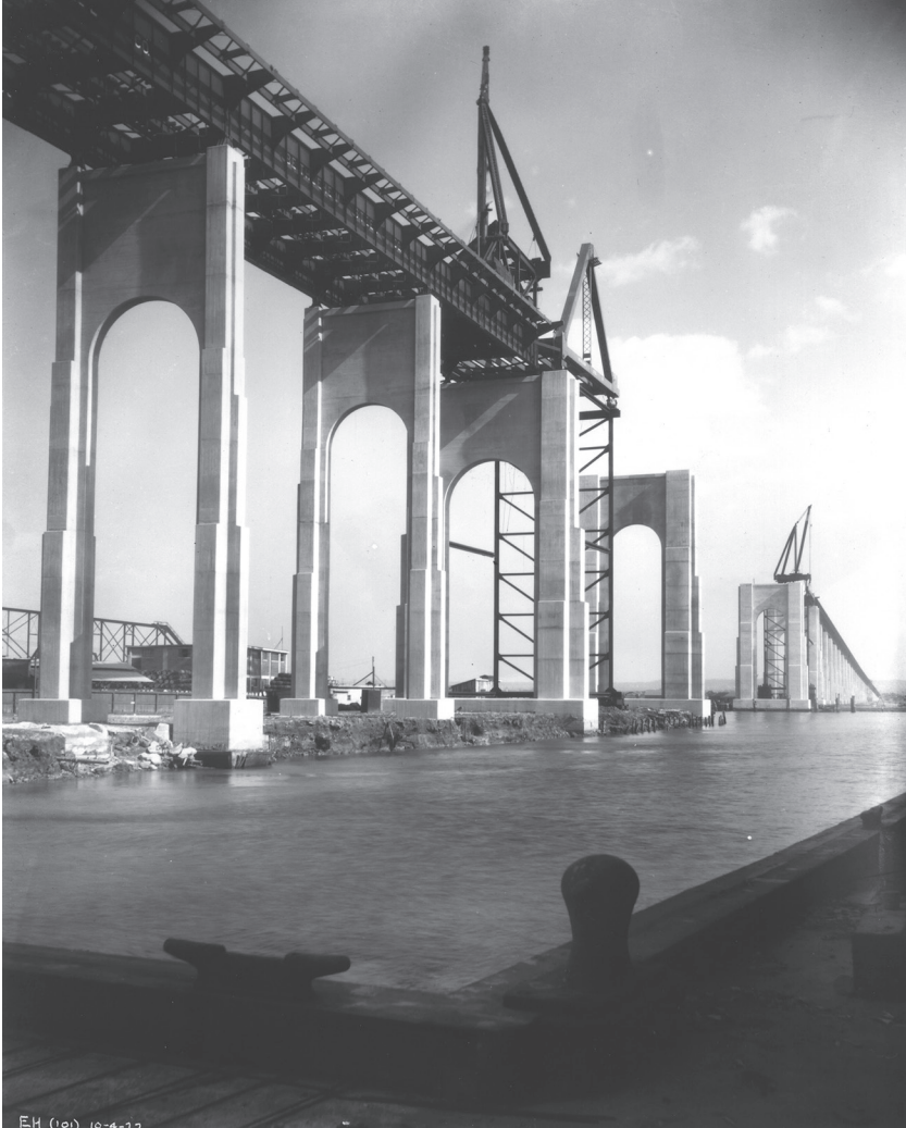
Fig. 7.2. Goethals Bridge construction.
