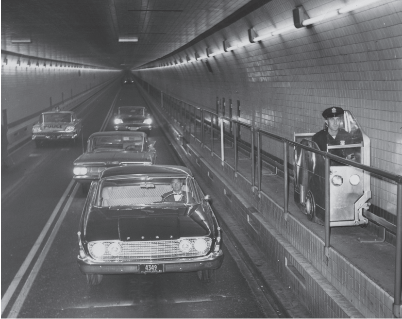
Fig. 10.3. Port Authority officer traveling in Lincoln Tunnel's catwalk car (1960). ( Photograph from the Lincoln Tunnel Collection, reprinted by permission of the Hoboken Historical Museum and the Port Authority of New York and New Jersey. )
