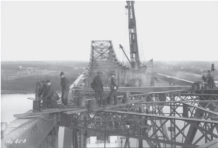
Fig. 7.1. Construction of the Outerbridge Crossing.
