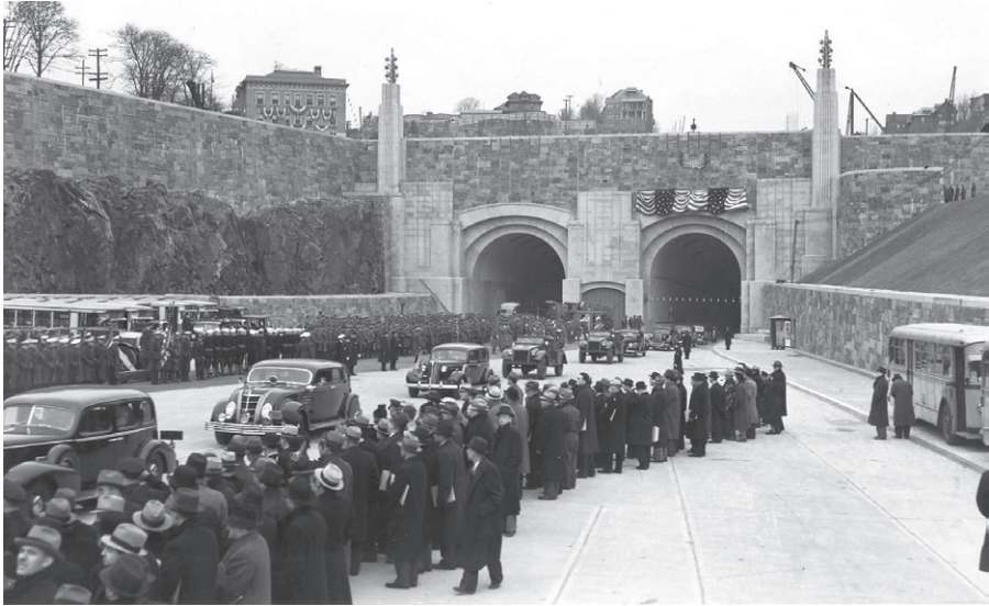
Fig. 2.8. The second tube of the Lincoln Tunnel opened in 1945. (Photograph reprinted by permission of Port Authority of New York and New Jersey.)
