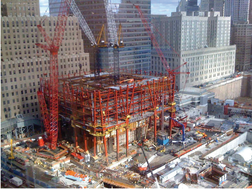
Fig. 8.8. Construction of One World Trade Center (Freedom Tower) in 2009. (Photograph by Westmc9th, December 2009. Courtesy Wikimedia Commons, CC BY-SA 4.0.)
