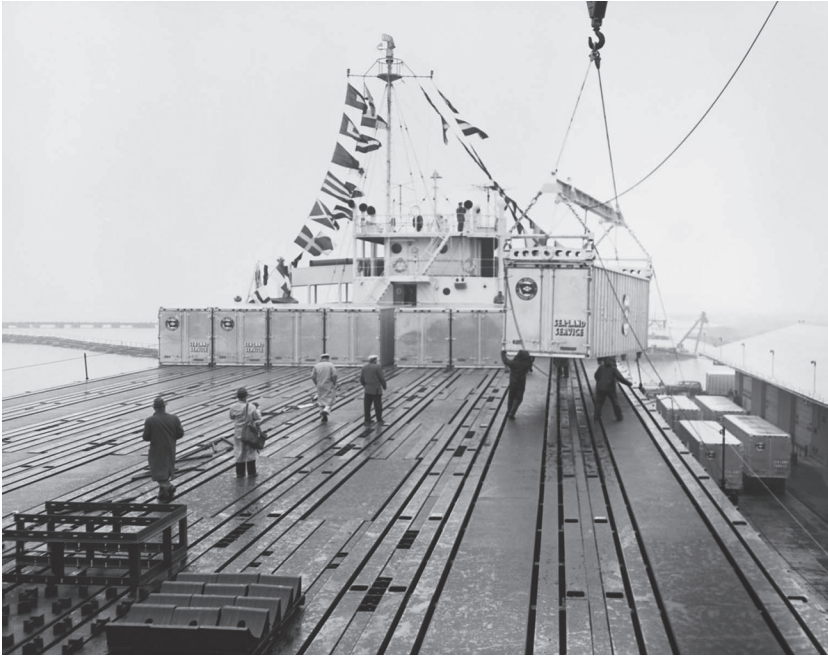
Fig. 4.4. Crane placing containers on the 1956 maiden voyage of the Ideal X in Port Newark, New Jersey.
