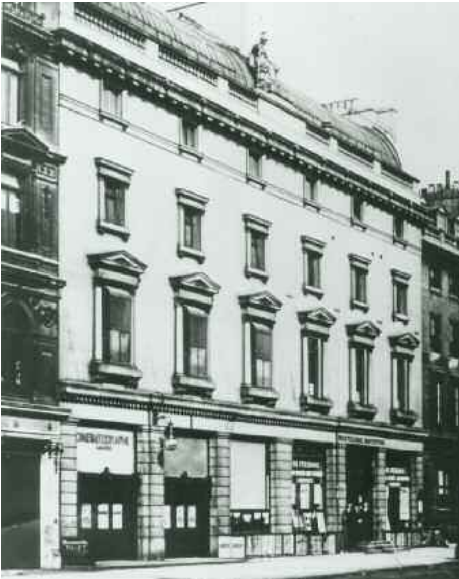
Fig. 7 The outside of 309 Regent Street in 1896. The current facade dates from 1910–12.
