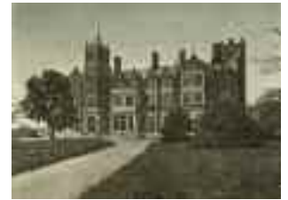
Fig. 1 Holly Hill House built for Quintin Hogg near Southampton, taken c. 1884. The house burnt down in July 1886.
