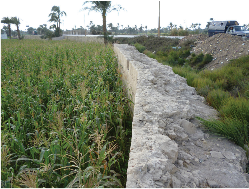
Figure 11. Stone-faced section of the Iṭṣā-‘Izbat Abū al-Nūr dike near Iṭṣā. Photo by author, 2011.
