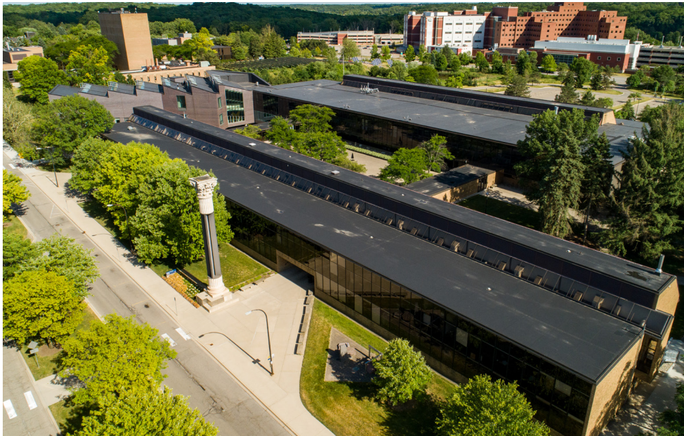
Art & Architecture Building | By Michigan Photography
