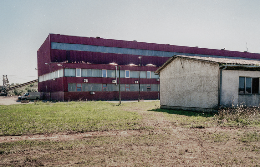
Figure 8. The main building and the infamous white house at Omarska mine near Prijedor, used as a camp in 1992. (Courtesy of Pawel Starzec.)
