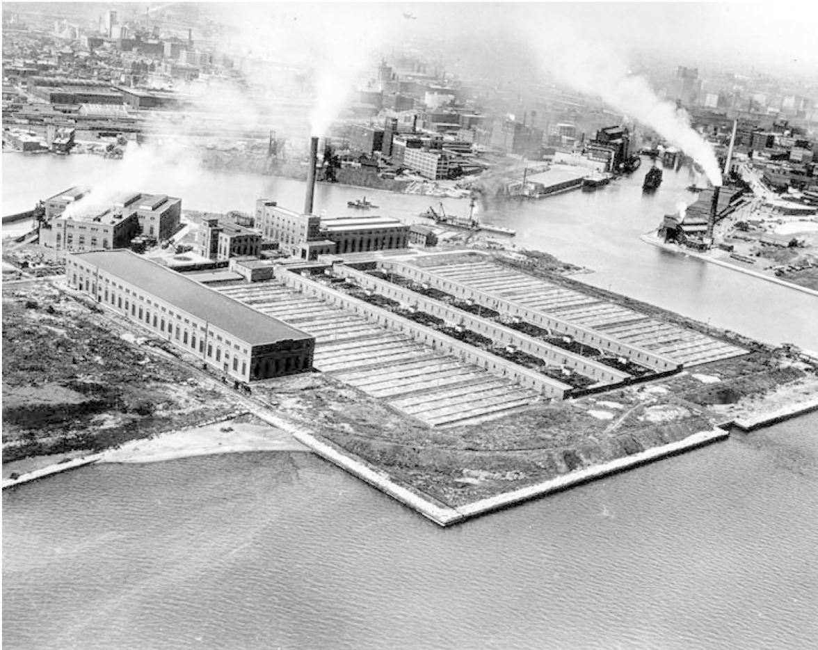
Figure 0.1 Jones Island Treatment Plant, Milwaukee Sewerage Commission, c. 1927. When this plant, located in Milwaukee's harbor, began operation in 1925, it was the largest sewage treatment plant in the world. Milwaukee had established a testing station there in 1915 that was instrumental in the development of the activated sludge process. The plant is still operating today. Source: Milwaukee Metropolitan Sewerage District
